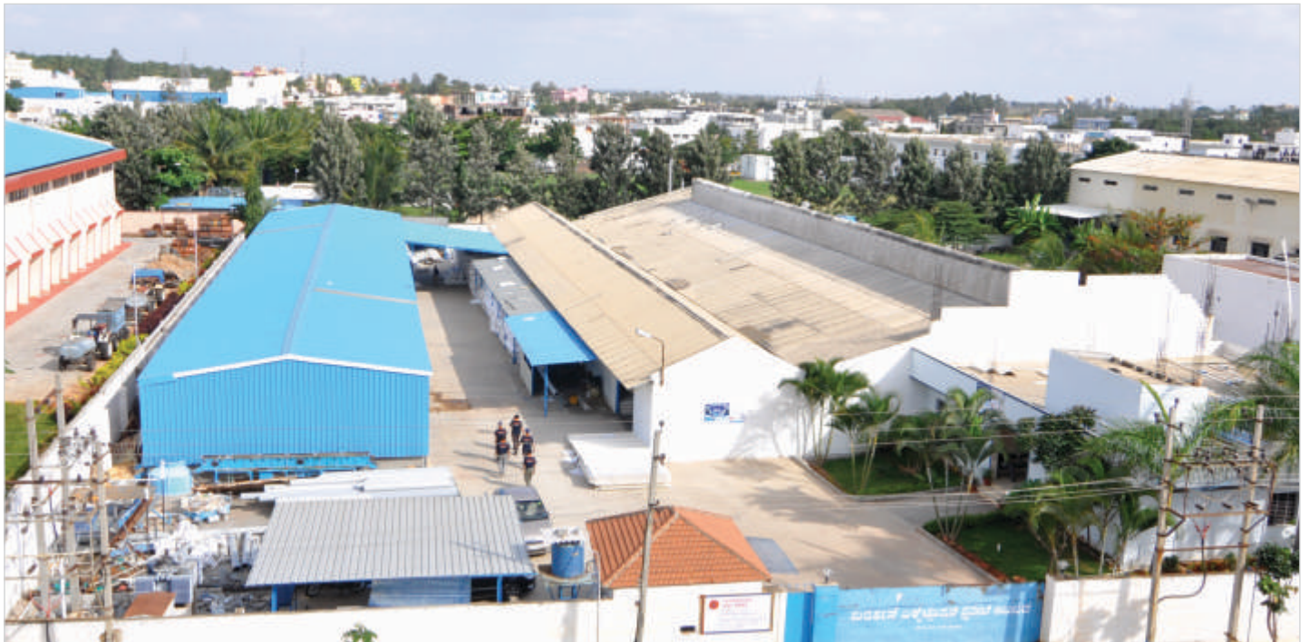
Factory view - Bommasandra Industrial Area, Hosur Road, Bangalore.
